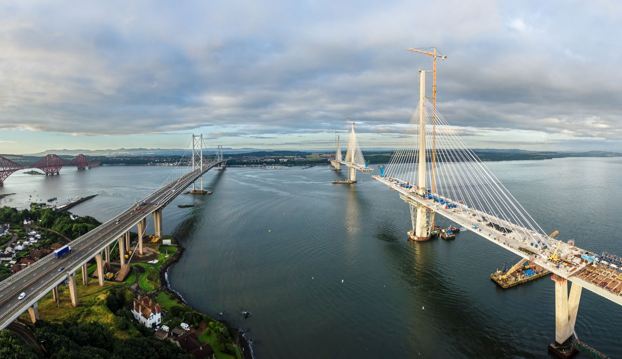
The Queensferry Crossing is one of the largest infrastructure projects in Northern Europe.
