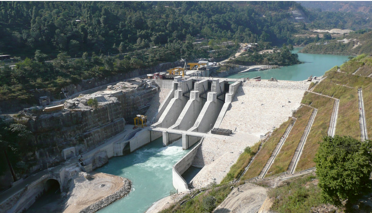
Hydroelectric power plant Middle Marsyangdi, Nepal
