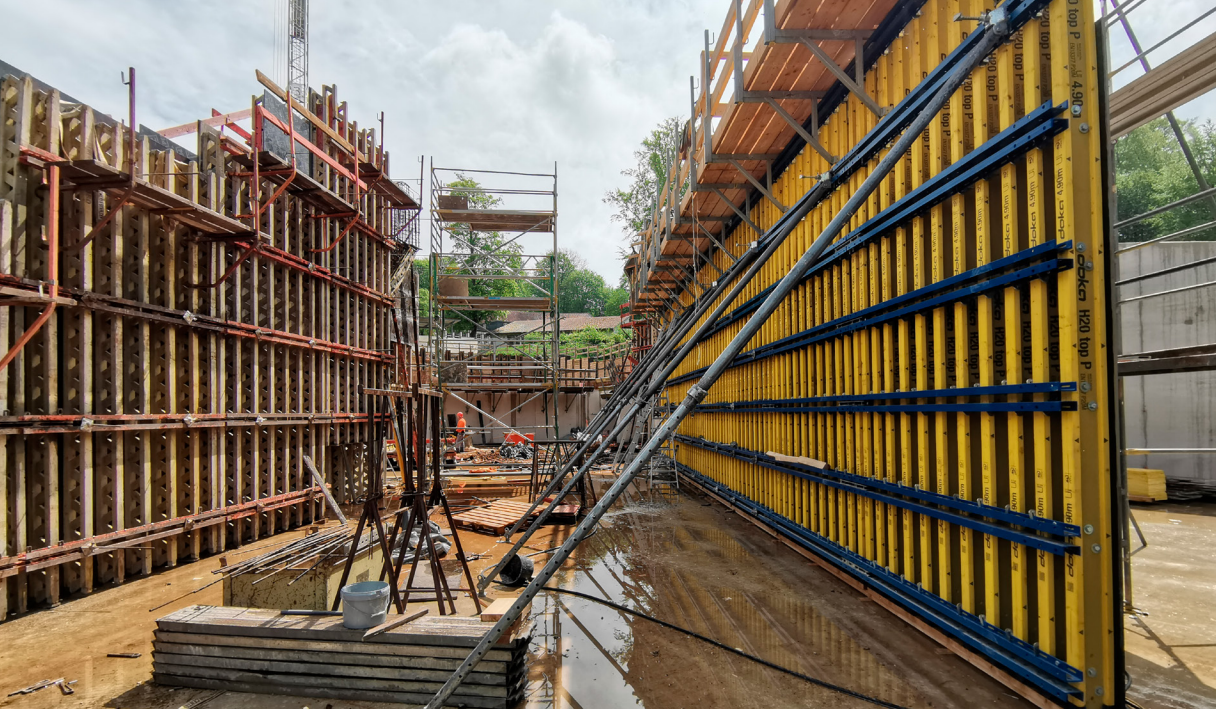
View of the construction site.
