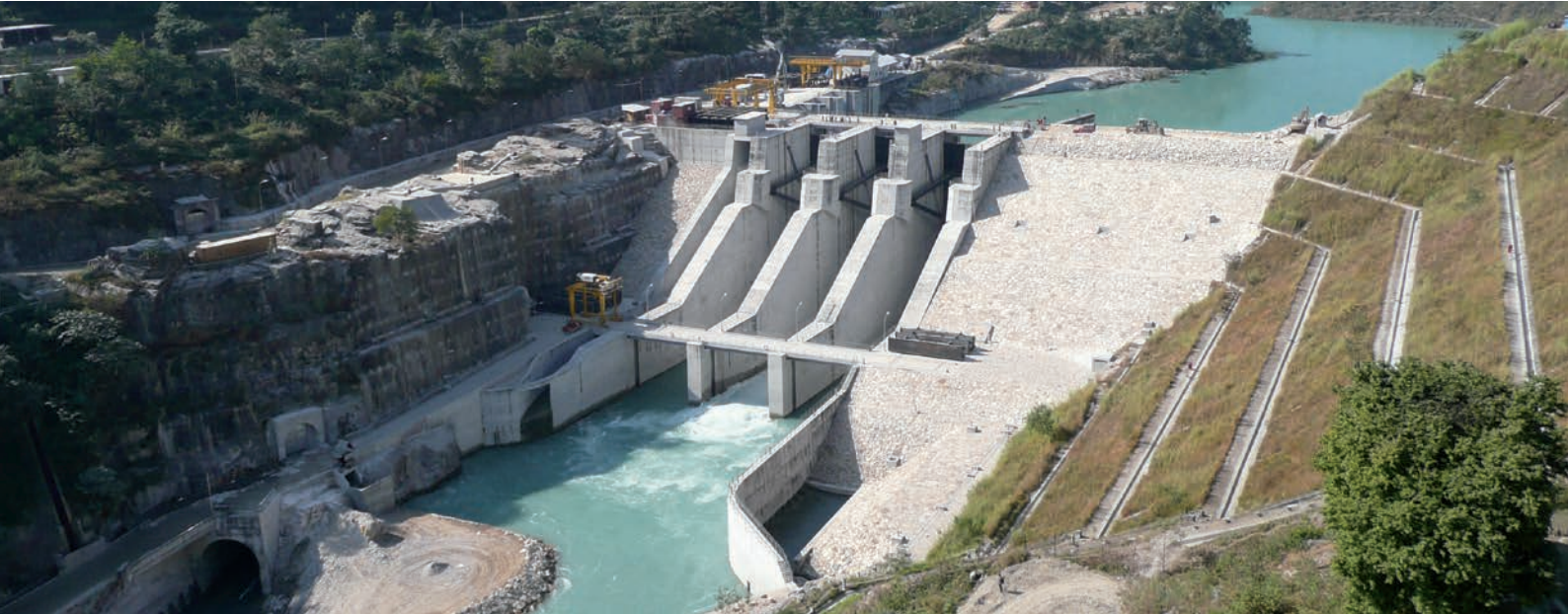
Project: Hydroelectric Power Plant Middle Marsyangdi, Nepal, Constructor DYWIDAG International GmbH
