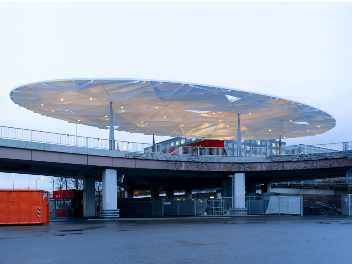
Messe Frankfurt – North Gate, oval roof on existing street bridge, Photo: Ingo Schrader
