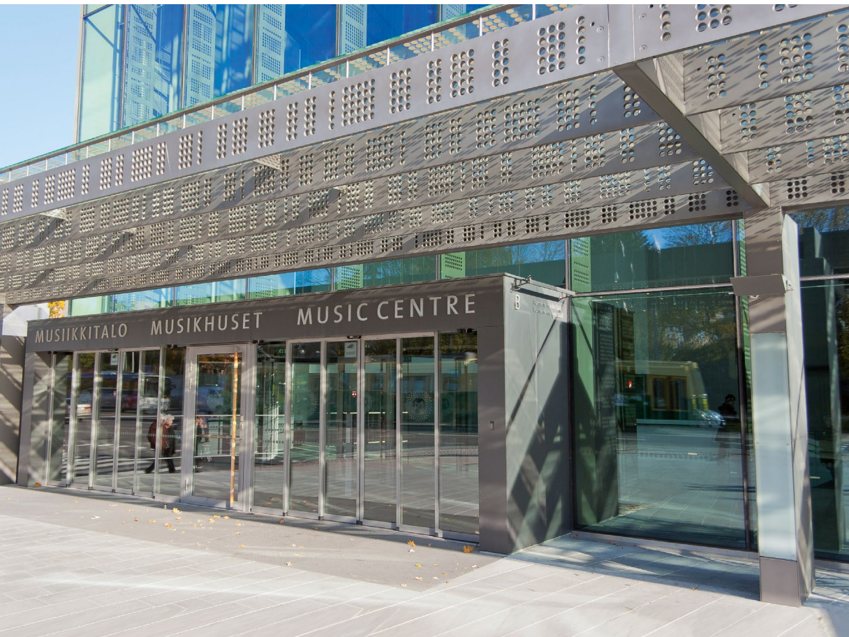
Helsinki Music Centre, Helsinki, Finland
