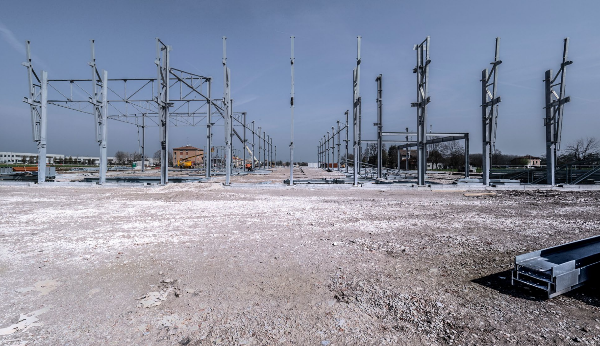
Installation of structural steel framework With courtesy of CSF Inox SpA and C&P Studio
