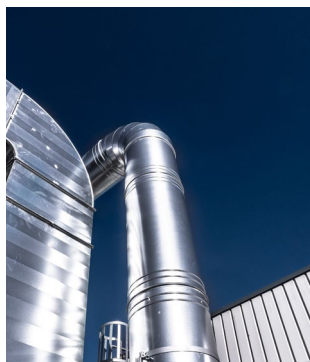
Left: Mounting the roof truss in the metal fabricators workyard Top right: Details of the air treatment plant Bottom right: Extraction systems in the open mid-level floor With courtesy of CSF Inox SpA and C&P Studio
