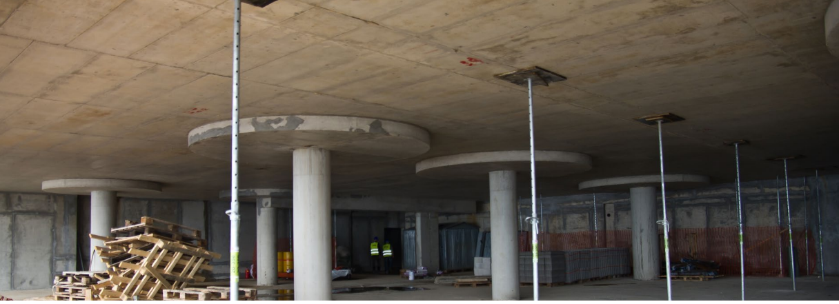
Picture above: View of the concrete ceilings with capitals in the restaurant area
