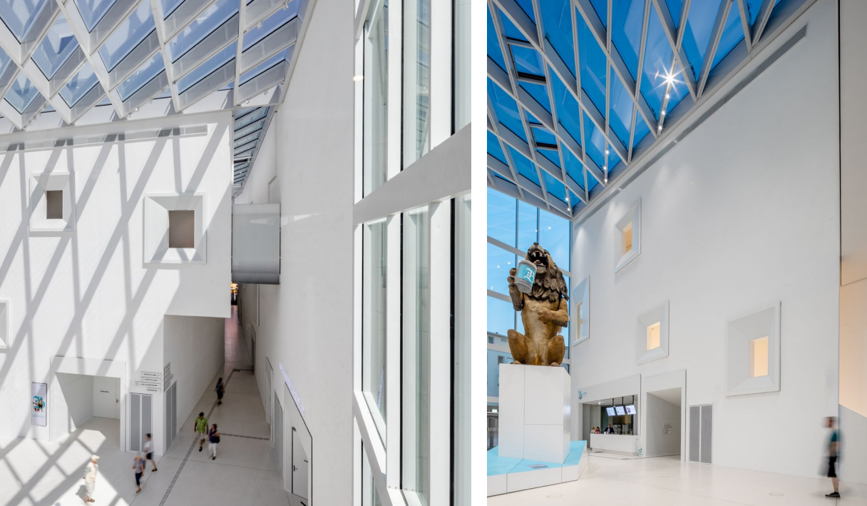
Interior view: Foyer flooded with light © wörner traxler richter planungs-gesellschaft mbh, Photo: Frank Blümner
