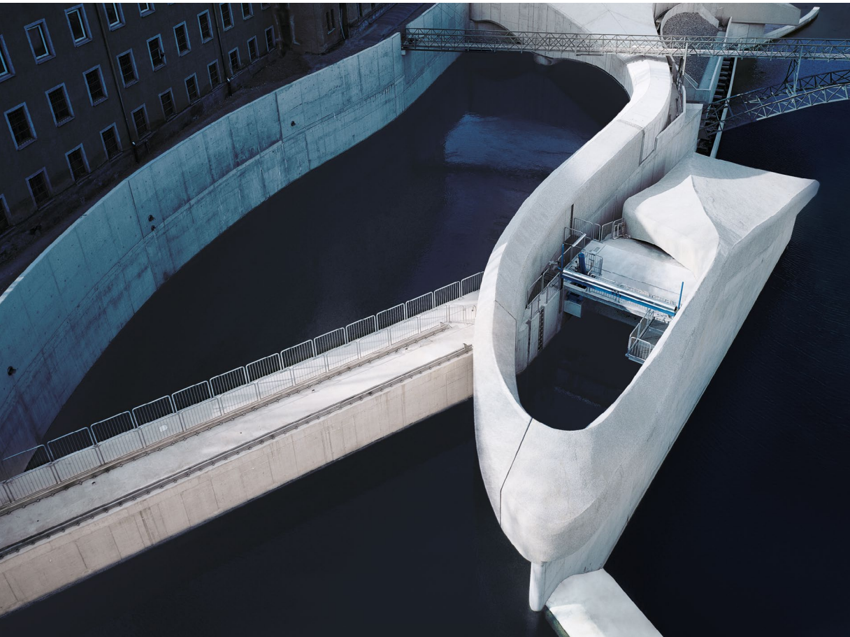
Keselstraße hydroelectric power station, Kempten
