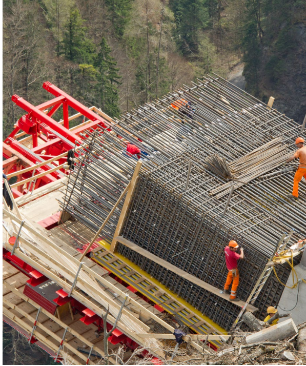
Valens: Reinforcement of the ground level arc;
