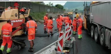
Patrick Zumbühl explains the structural engineering features of the A2 repair: "The existing surface of the northern and southern lanes will be replaced completely and strengthened by means of milling and resurfacing. The existing longitudinal slope is between a 0.25 and 0.7 percent gradient, and therefore places high demands on the accuracy of the installation of the new road surface." He was able to meet these needs as efficiently as possible using the Allplan Highway module.
