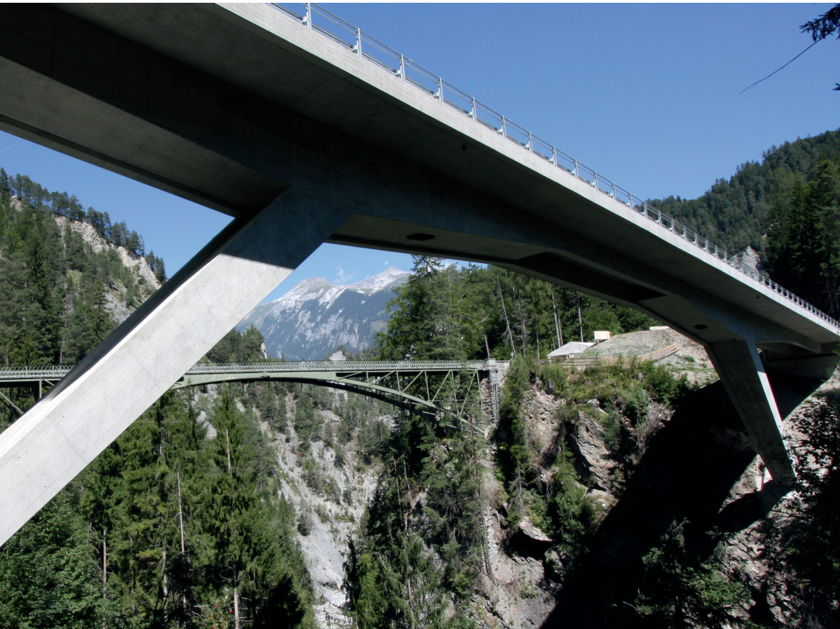
Versamertobel Bridge, Graubünden Canton, Switzerland
