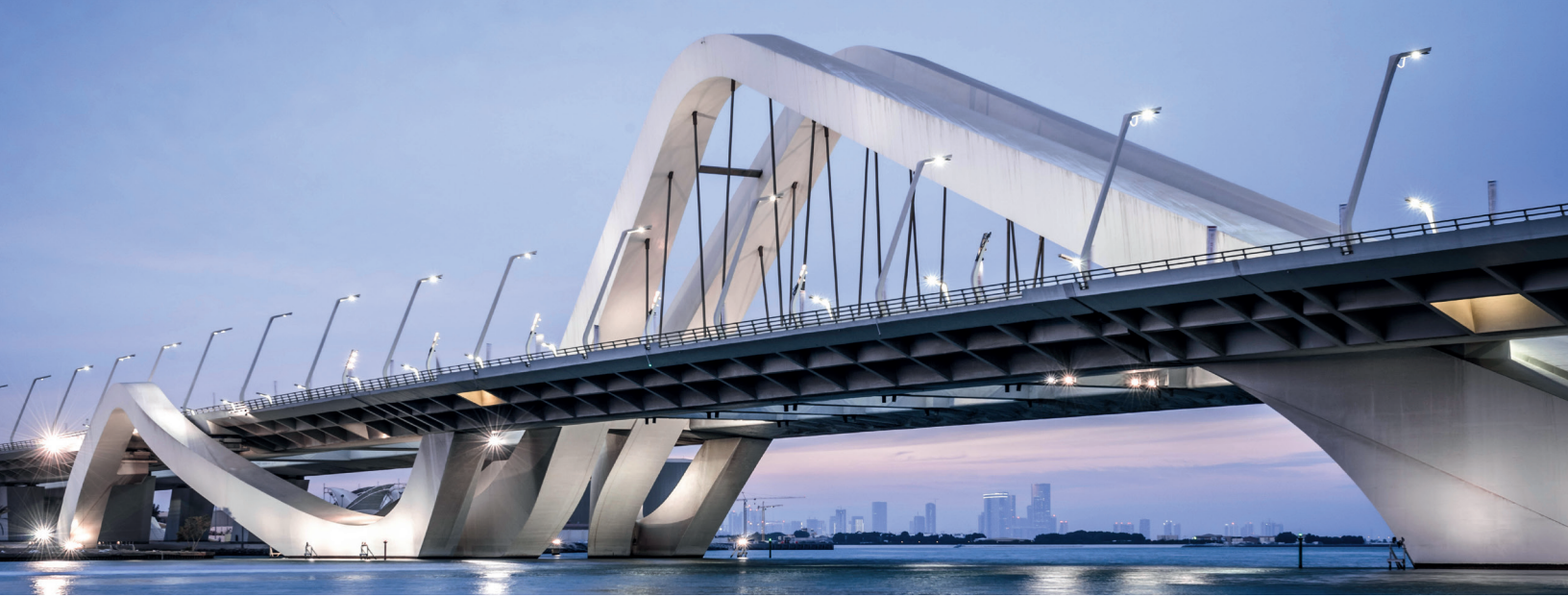
© Project: Sheikh-Zayed-Bridge, Abu Dhabi | © iStock | © photo: Richard Sharrocks
