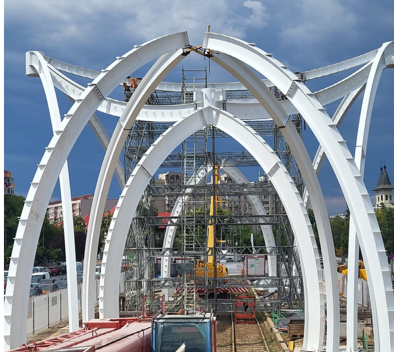
Temporary supports and on-site welding ensured stability and precision during the installation of over 600 unique canopy elements – all completed within a three-month construction window.
