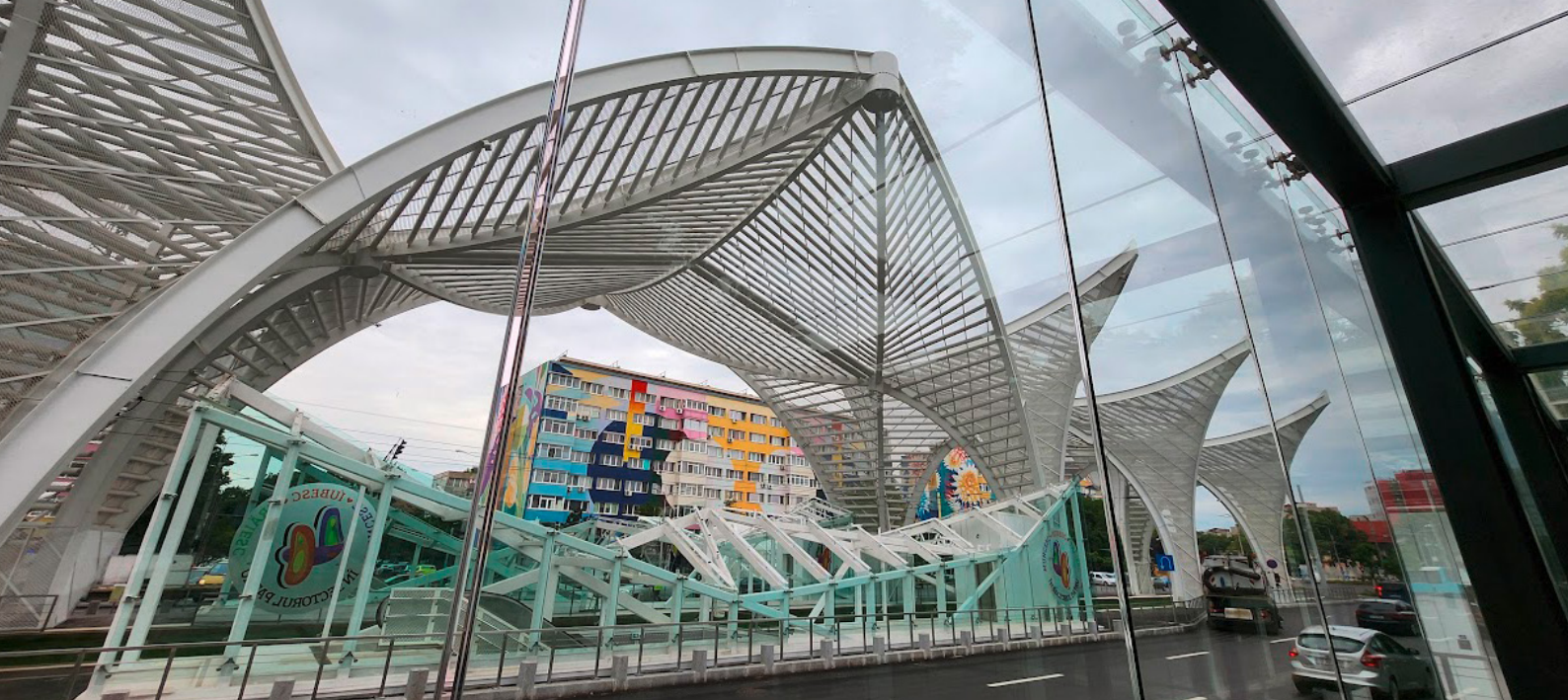
The completed Gate of Heroes canopy. The sculptural steel structure now serves as a visual landmark and multimodal transit hub for the area.
