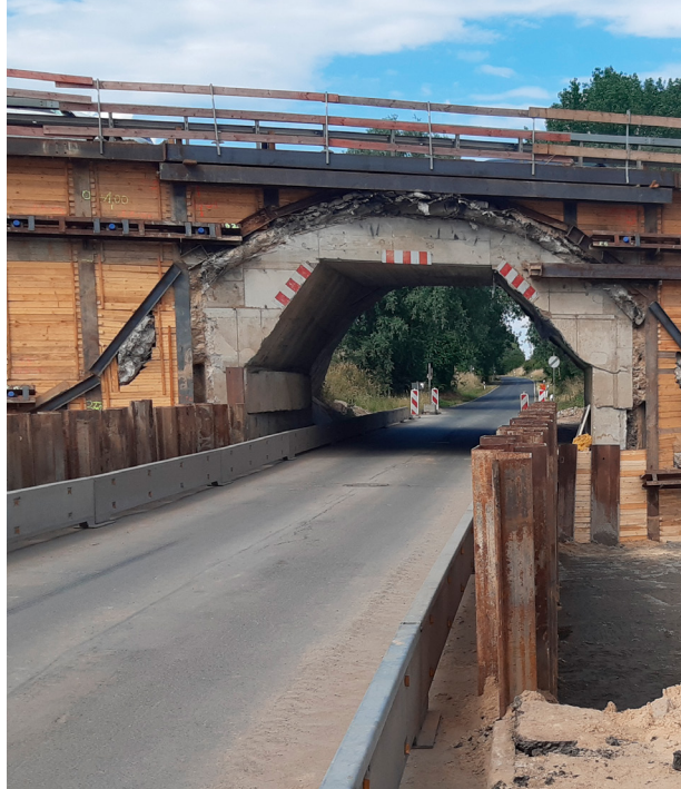
Havelland freeway construction site
