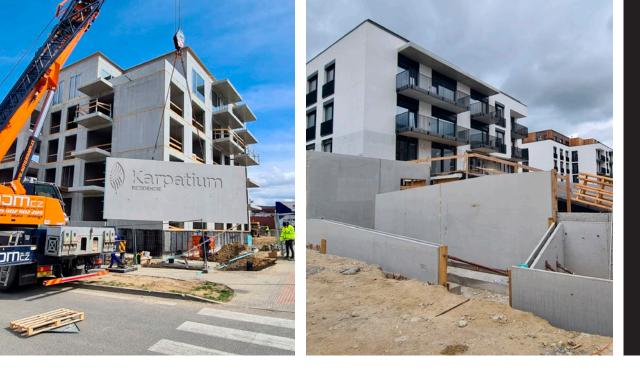
For the Karpatium Rezidence housing complex in Bratislava, the contractor relied entirely on precast elements and used prefabricated balconies, stairs, element slabs and double walls.
