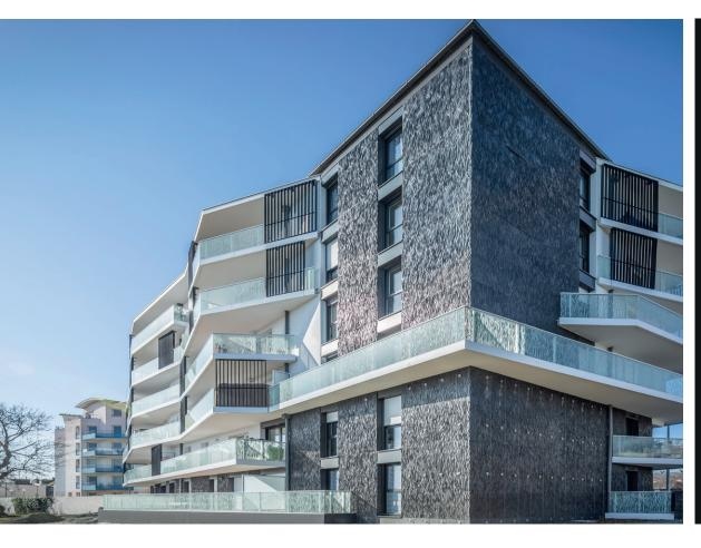
Precast concrete walls radiate liveliness with the help of structural matrices
