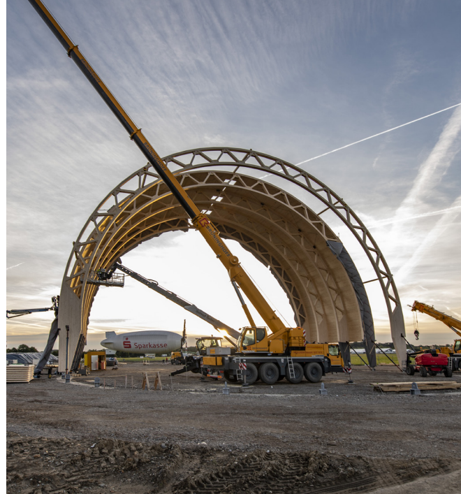
A total of 557 tons of spruce wood from local forests was used. This saved approx. 156 tons of CO 2 .
