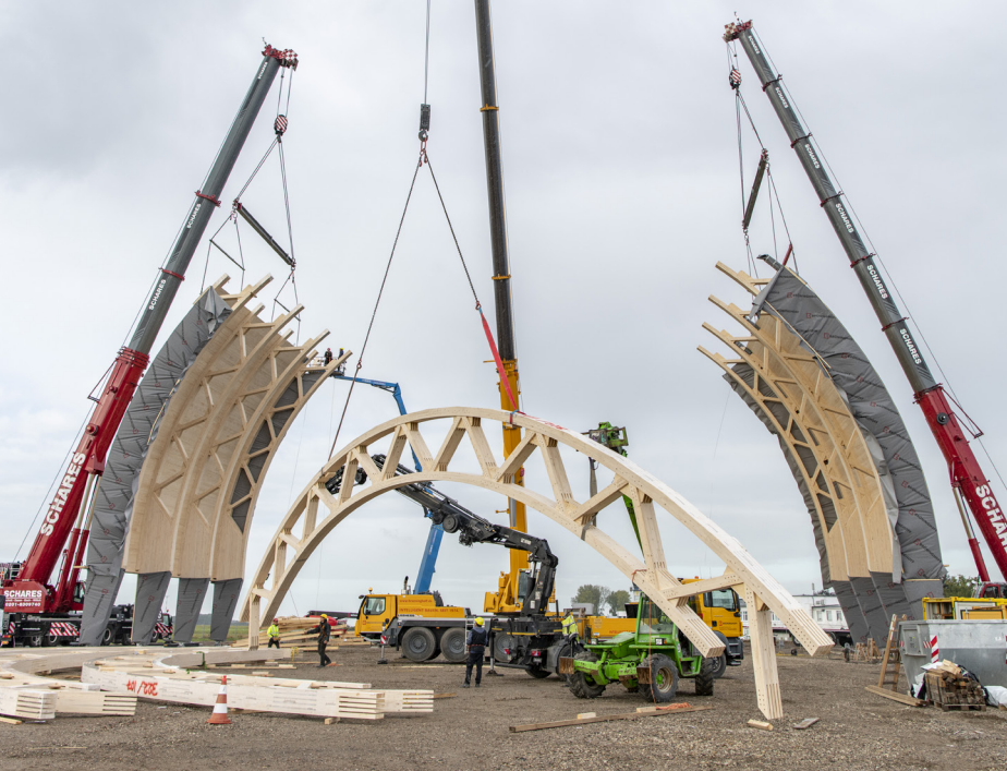
The airship hangar's 100% wooden supporting structure consists of 15 two-hinged arches, each 26 meters high.
